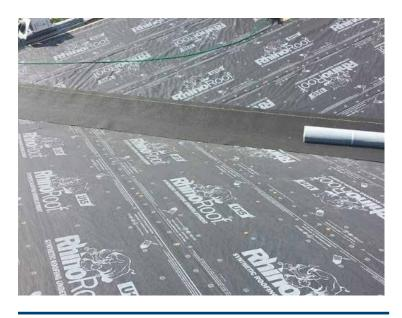
We install ice and water shield in the valley's for extra protection.
