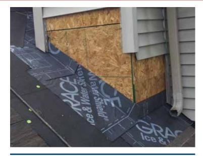
Chimneys are one of the most common areas that leek on a roof. We install ice and water shield around the chimney as extra protection to help prevent this problem.
