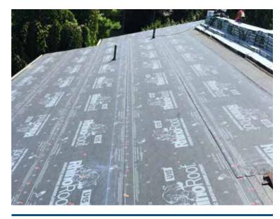
We dry the entire roof in for protection from the rain before we begin installing the shingles.
